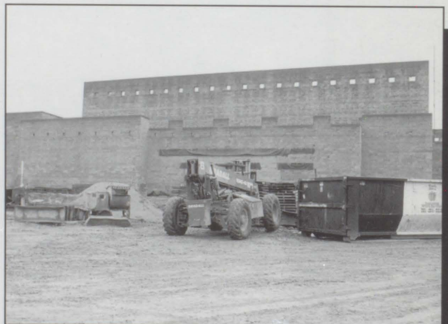
2004 Additions Under Construction
